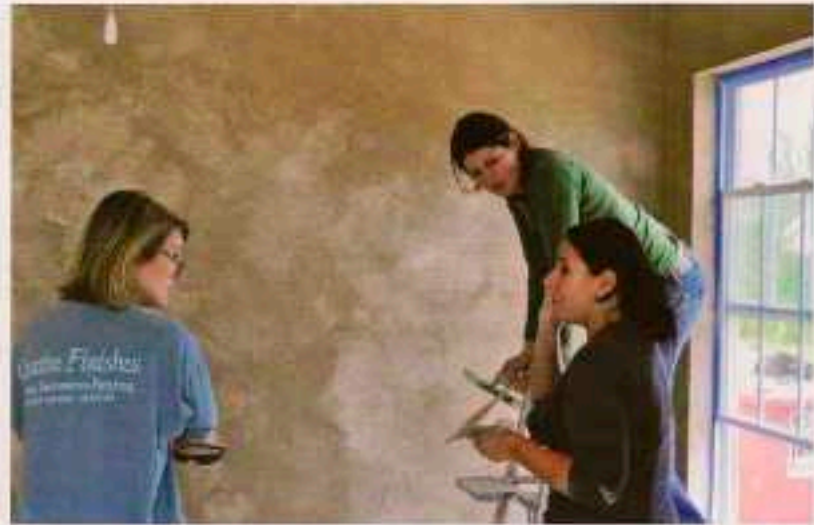
Volunteers work on the living room finish.
